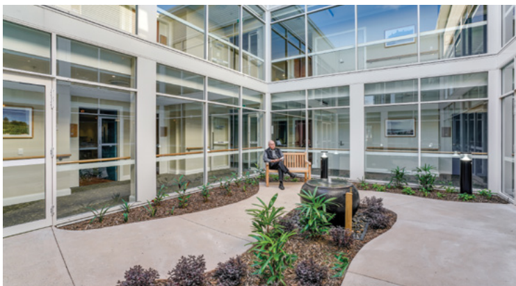
Construction of our Charles O'Neill Home in Mayfield West is complete – July 2020
